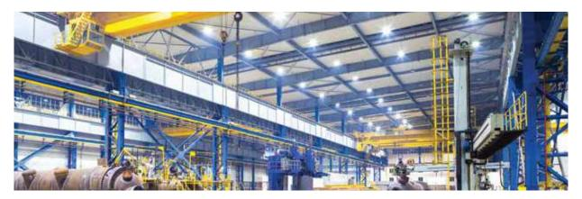
As their name implies, high-bay lights are used to illuminate spaces with high ceilings. That usually means ceilings ranging from 20 feet to approximately 45 feet. Low-bay lights, on the other hand, are used for ceilings 20 feet and under. Because a high-ceiling location has more space to fill, a high-bay by definition is a powerful light source that can brighten up a large area.
